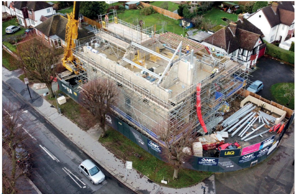
Haling Park Road, Croydon
